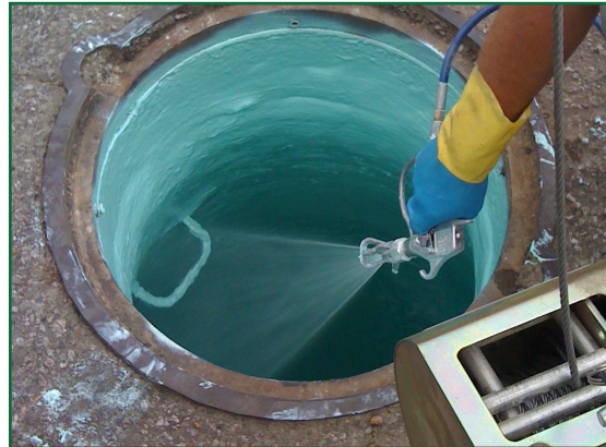
Novocoat SG2500 high build epoxy application.
