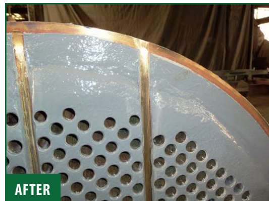
Tube sheet resurfaced using Novocoat EP5720 Ceramic Paste.
