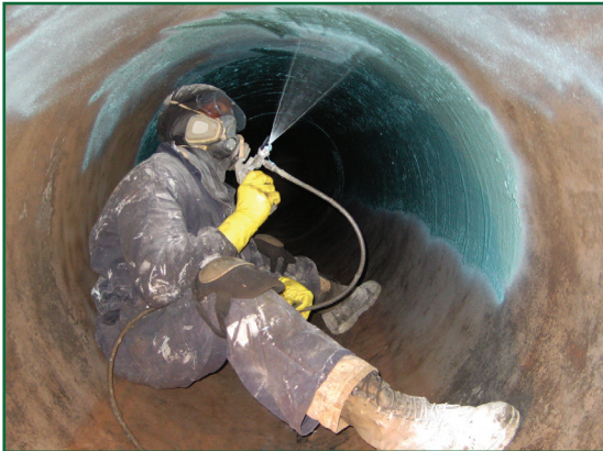
Novocoat SG2500 high build epoxy application.
