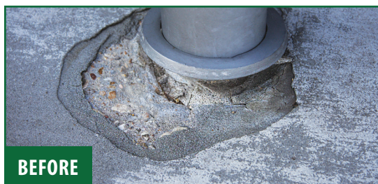
Novolite Repair Mortar used on concrete.
